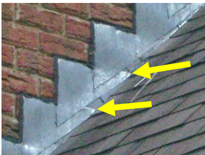
Upper edge of flashing exposed
