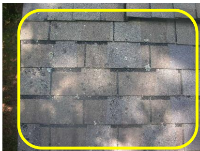
Black dots are dime sized areas of missing granules on porch roof
