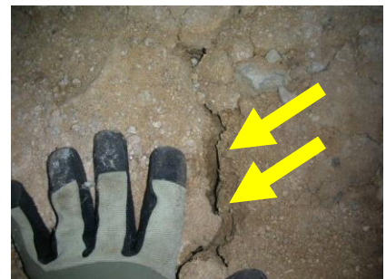
Finger width cracks in crawlspace soil under exterior living room foundation wall
