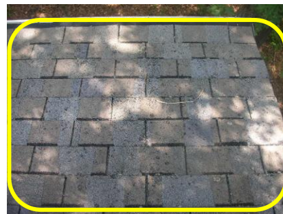
Black dots are dime sized areas of missing granules on porch roof
