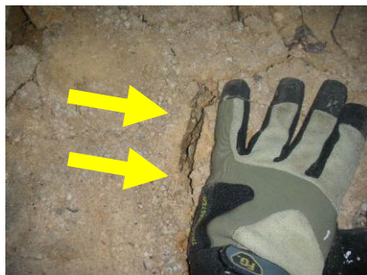
Finger width cracks in crawlspace soil under exterior living room foundation wall
