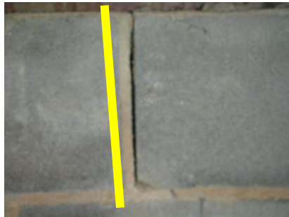
Crack in front foundation wall under living room
