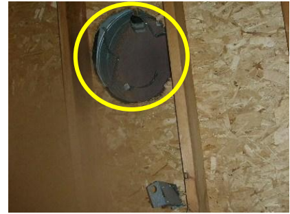
Attic fan removed
