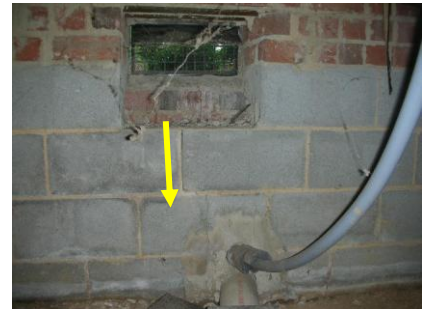
Crack in front foundation wall under living room
